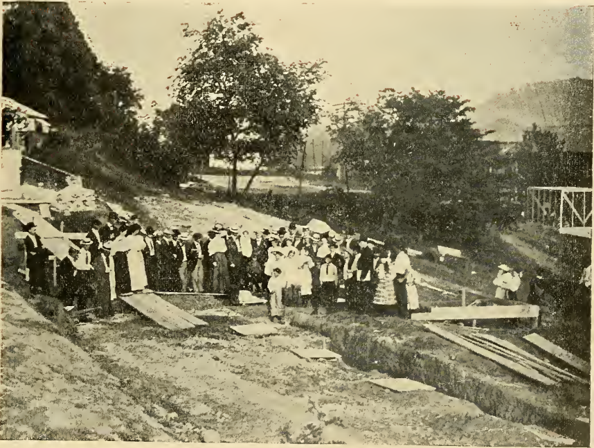
LAYING THE FIRST BRICK IN THE NEW AGRICULTURAL BUILDING.
